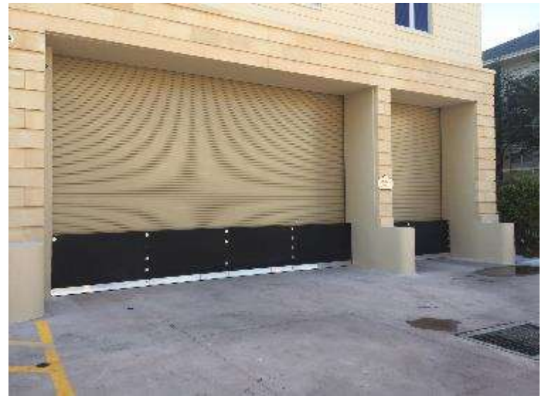
Flood Panel installed on Industrial garage in Tampa, FL
